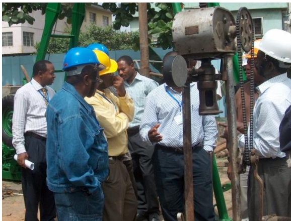
Fig. 5b: Typical Drilling For Onshore Geotechnical Investigation
