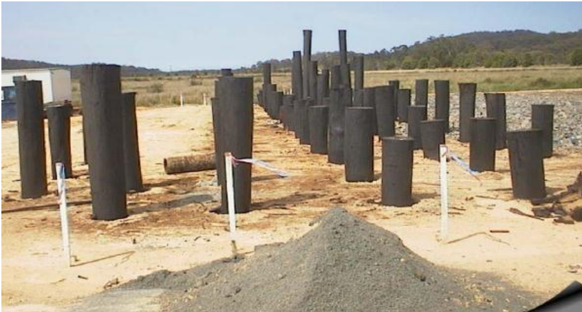
Fig. 10b: Deep Foundation (From Shah, A.)
