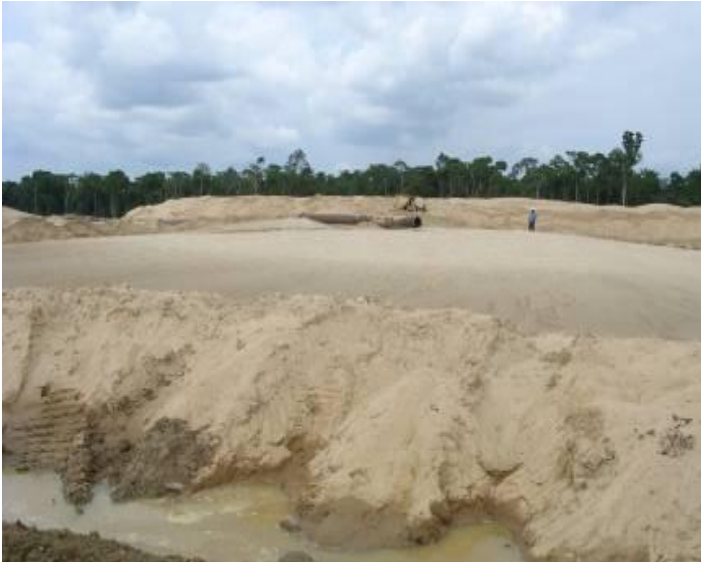
Fig 4.0: Dredging and Sand filling
