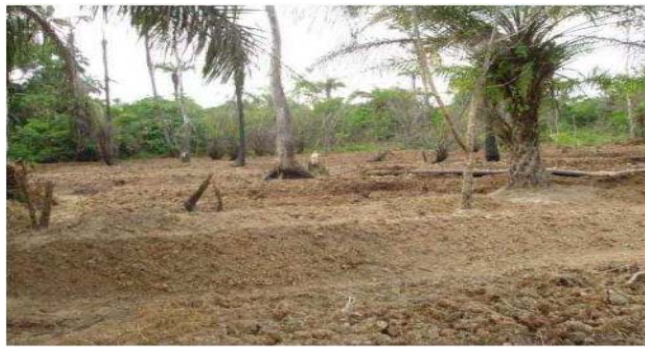
Figure 7.30b: Windrows constructed at polluted site
